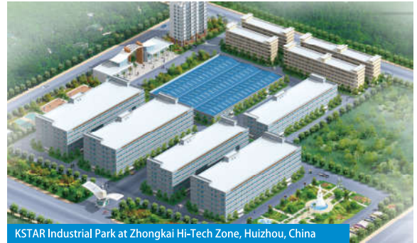
KSTAR Industrial Park at Zhongkai Hi-Tech Zone, Huizhou, China
