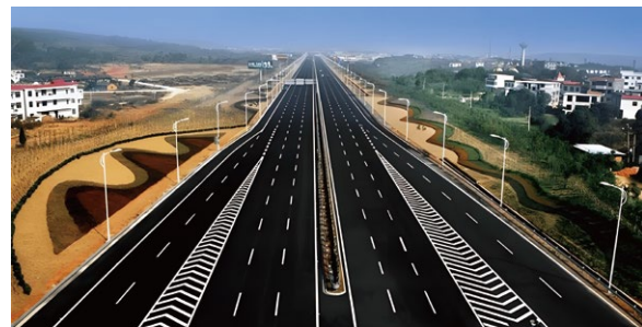
Ruili to Menglian Expressway Electromechanical Project
