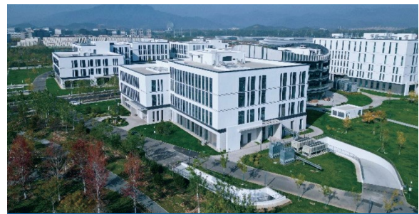
Peking University Biomedical Imaging Technology Cluster Large Facility
