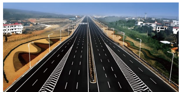
Ruili to Menglian Expressway Electromechanical Project
