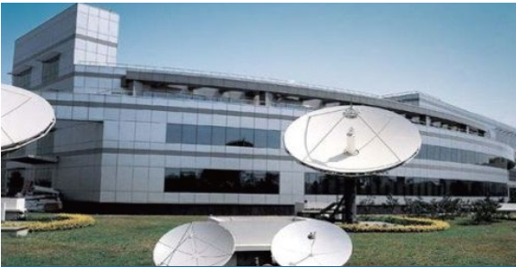
Shanghai Securities Waigaoqiao Earth Station
