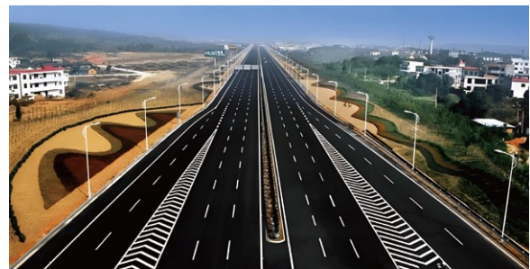
Ruili to Menglian Expressway Electromechanical Project
