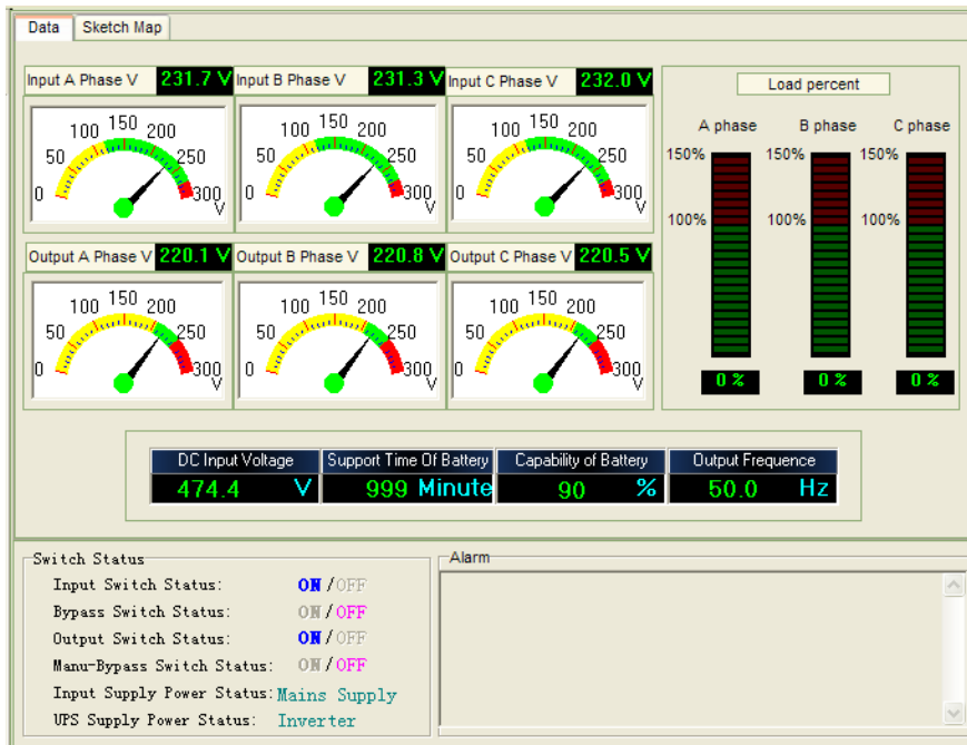
This figure displays partial current data of monitor UPS with meters.
